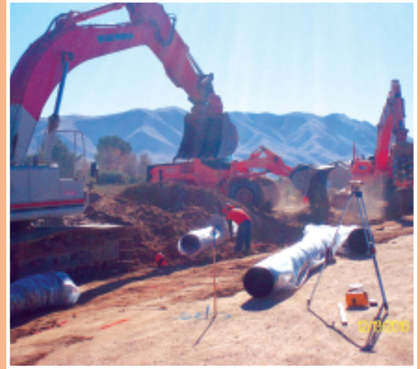
Pictured at right: Mockingbird Pipeline Installation
